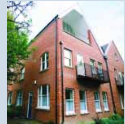
The exterior at 15 Sundridge Avenue
